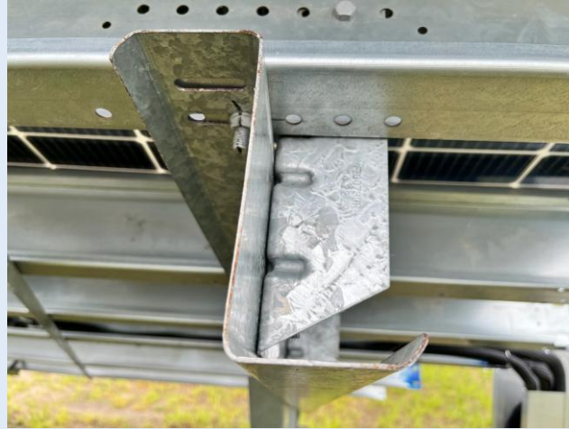
1.8-mm Z-shaped Channel Section on Fixed-tilt PV Frame
