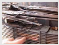
Transformer winding failure
