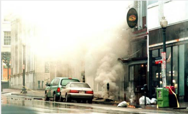
Cable replacement and upgrading
